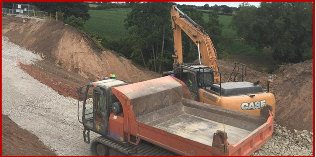
Diggers at Middlewich breach
