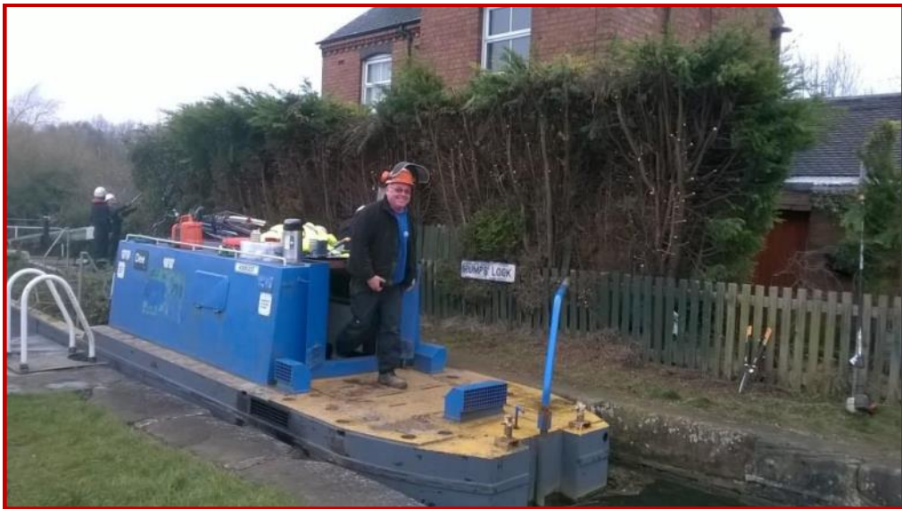
Vegetation clearance At Rumps Lock
