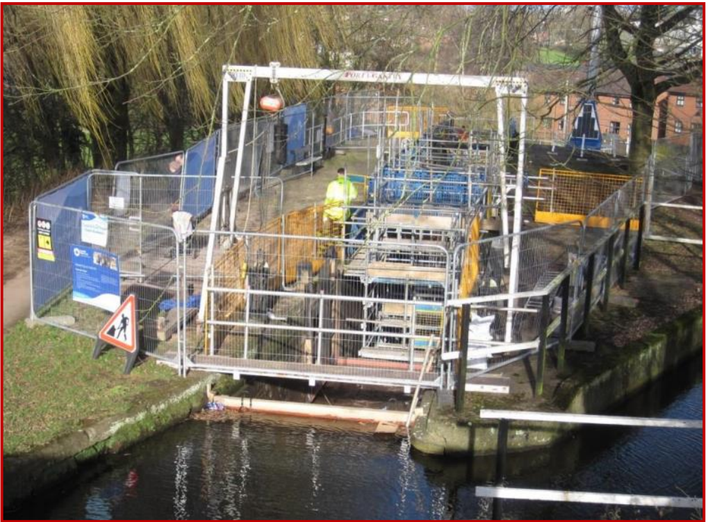
The staircase from the bridge above
