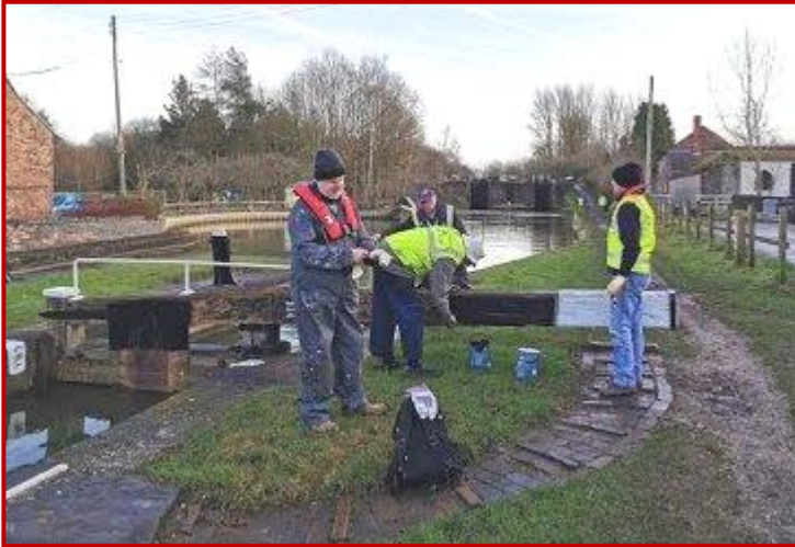
Painting Top Balance Beam on Lock 65 Photo Jane Har greaves
