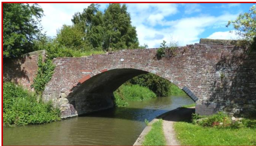
Bridge Nine Showing parapet damage
