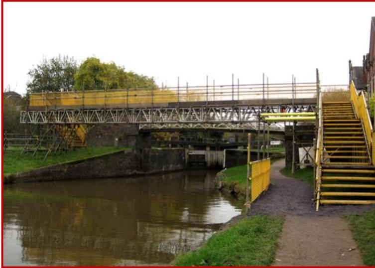
Here is the temporary structure allowing residents to cross the canal safely (and making it much easier for single-handed boaters to work through the lock).
