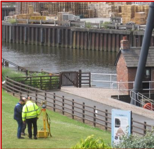
Measuring with theodolite Preparatory to repairs
