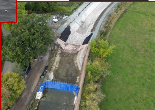
Aerial view of the final 10 metres
