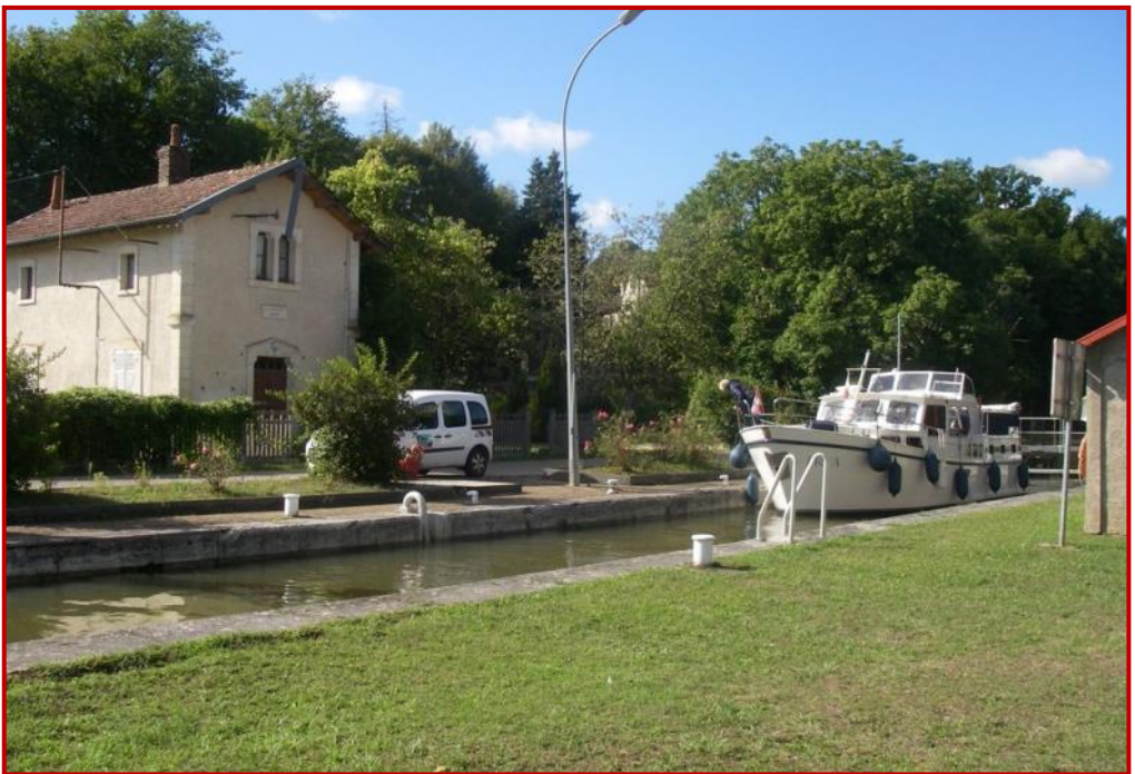
Cruiser entering the replacement locks
