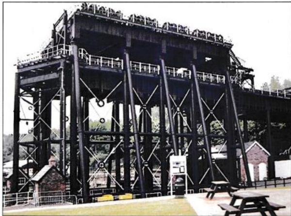
The reopened Lift in 2002, before its official reopening in 2003. (Photo: William Rowley)
