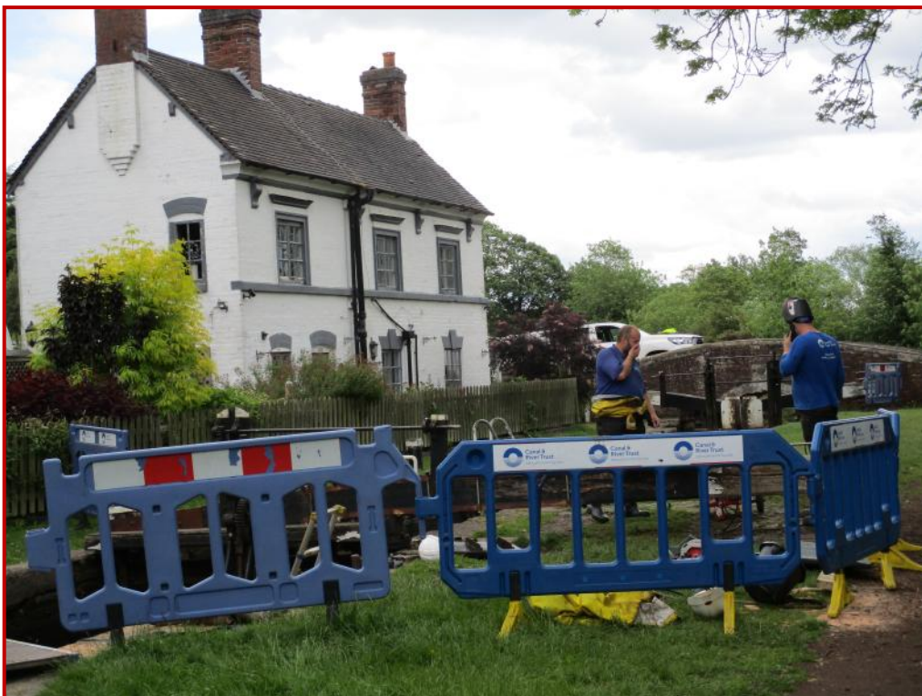
Colwich Lock Repair (P5)
